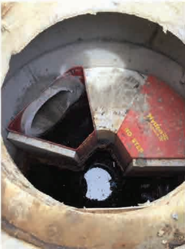
Hydro-seperator in chamber 1
