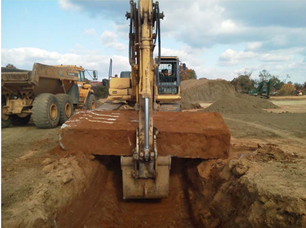
Figure 28 - Concrete Slab Causing Anomaly, Part of Navy Annex Foundations (Schneider 2013)
