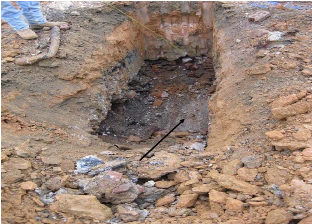
Figure 29 - Remains of Concrete Foundations of Quarters K Dining Hall Cause of Anomalies (Schneider 2013)
