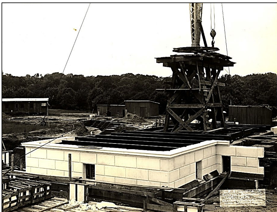
Figure 18: Crane Used to Install Marble, Arlington Memorial Amphitheater (October 1915) Source: Historical Research Collection, Arlington National Cemetery
