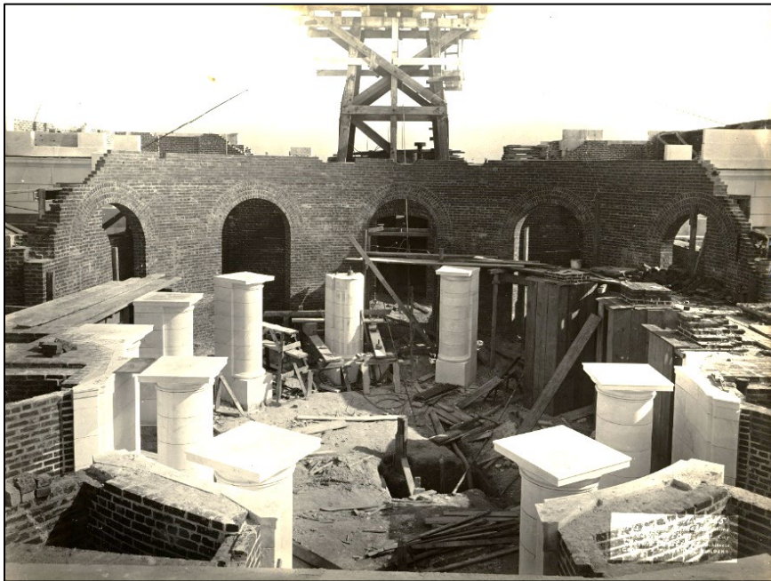
Figure 19: Installation of Chapel Columns (November 1915) Source: Historical Research Collection, Arlington National Cemetery
