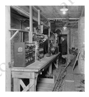
Figure 9.17. In addition to the loudspeakers, AT&T also installed equipment under the Amphitheater to amplify the microphone placed on the apse of the amphitheater. (*Library of Congress*)
