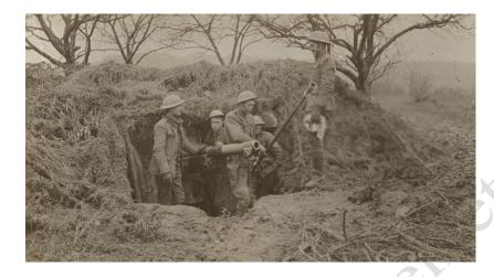
Figure 3.1. American artillerymen photographed with a French made 75mm field gun which revolutionized modern artillery during World War I. Its rapid-fire system allowed gunners to unleash up to 15 aimed rounds per minute without re-aiming, saturating the enemy with shrapnel and high-explosive shells. The weapon's unprecedented rate of fire made it a key driver of the war's horrific mass casualties. (National Archives)
