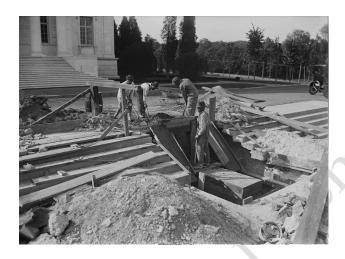
Figure 8.9. Workers prepared the site on the east side of Memorial Amphitheater to accommodate the crypt and the placement of the Tomb's base. This construction work began in mid-October 1921, just about one month prior to the Unknown's funeral. (*Library of Congress*)
